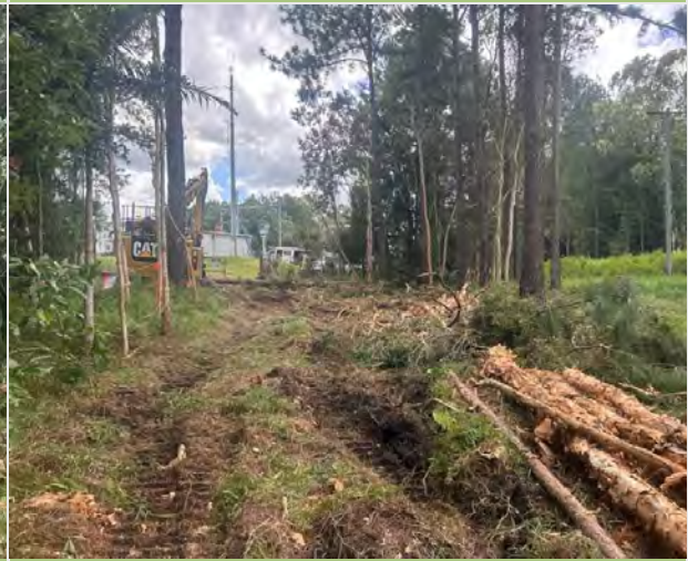
Figure 7. During Clearing Works:
