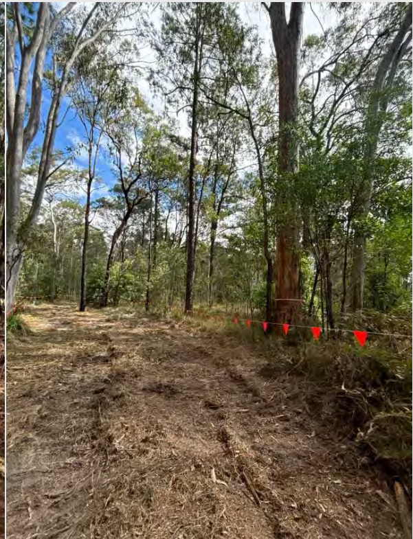
Figure 5. Post Clearing Works: SI Clearing extents vegetation clearing and mulched
