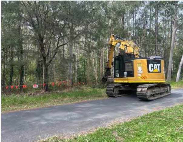
Figure 2. During Clearing Works: Excavator with grooming head
