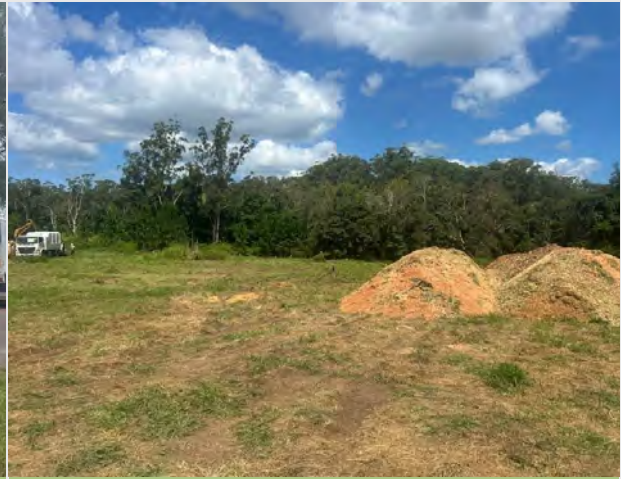
Figure 5. During Clearing Works:
