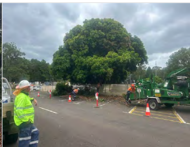
Figure 3. During Clearing Works:
