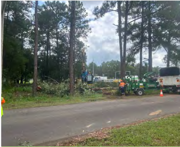
Figure 4. During Clearing Works:
