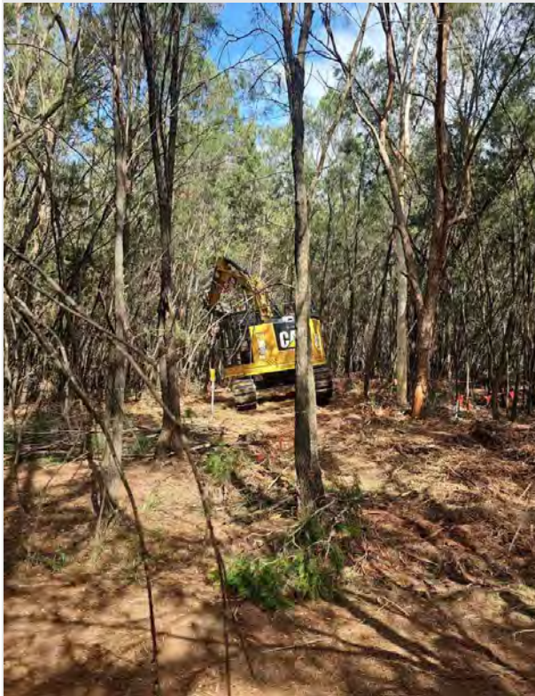
Figure 4. During Clearing Works:
