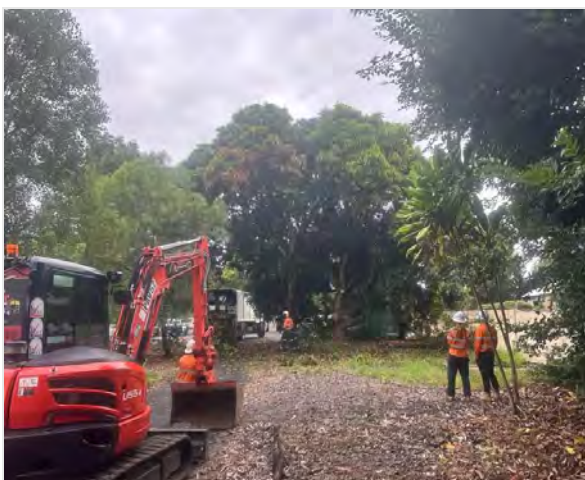
Figure 2. During Clearing Works:
