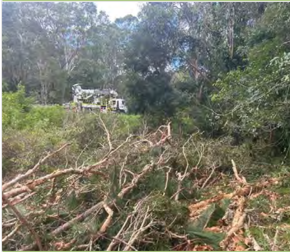
Figure 6. During Clearing Works:
