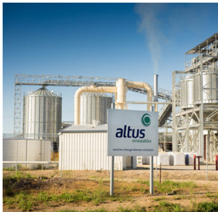
Altus Renewables production plant at Tuan (photograph courtesy of Altus Renewables)
