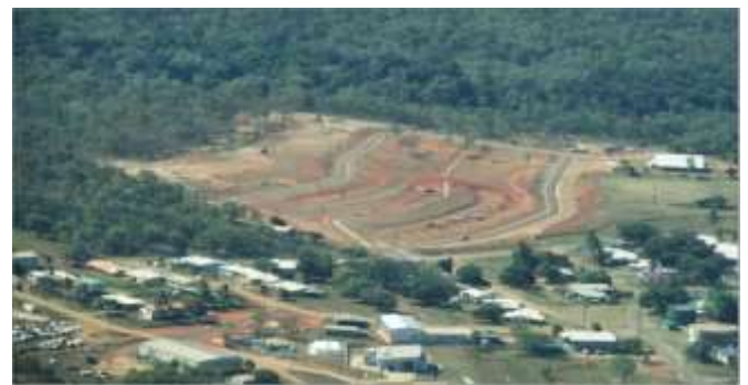
Work being undertaken to deliver infrastructure.
