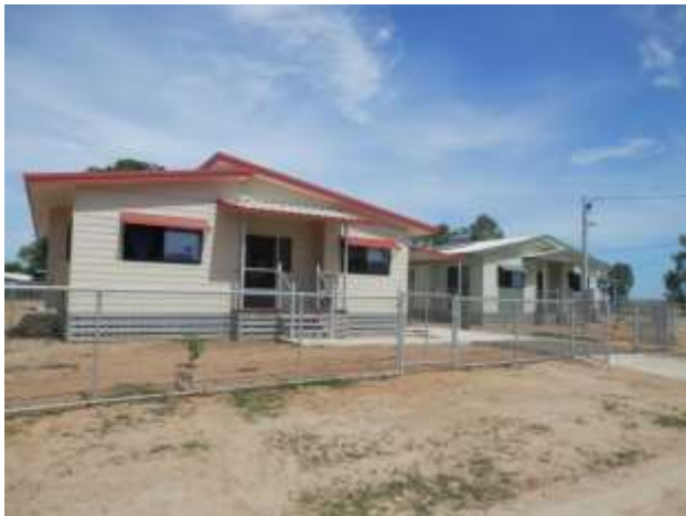
FK Gardner houses in Kowanyama finished and ready for tenants. (Photograph: Ian Anders, DATSIP).
