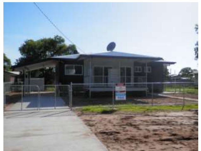
One of the houses constructed by the Pormpuraaw Aboriginal Shire Council. (Photograph: Ian Anders, DATSIP).
