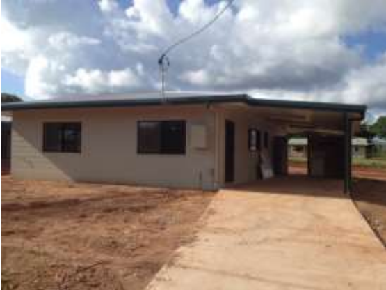
A new three-bedroom house finished and ready for tenancing. (Photograph courtesy of the Hope Vale Aboriginal Shire Council).
