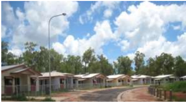
New housing construction has provided local employment opportunities in Aurukun. (Photograph: Garry Bailetti, DATSIP).
