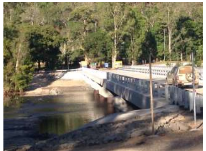
The completed Bloomfield River Bridge links to the Cook and Douglas Shire regions. (Photograph: Petrina Villaflor, DATSIP).
