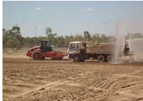
Construction work in subdivisions is well underway.
