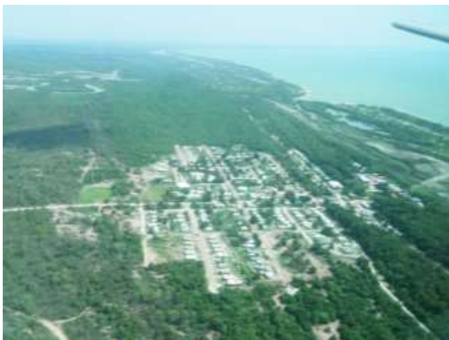
Completed FK Gardner houses prior to tenanting. An aerial view of the community of Pormpuraaw. (Photographs: Ian Anders, DATSIP).
