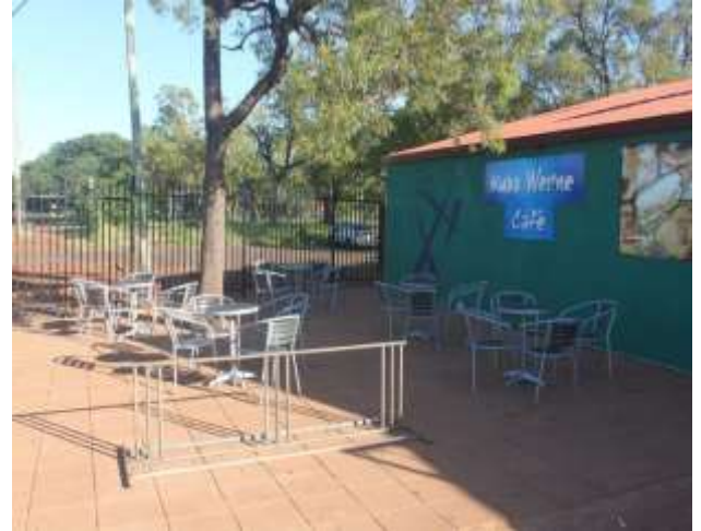
The new entry and courtyard area welcome diners to the Kuba Werne café (Photograph: Ian Woolford).
