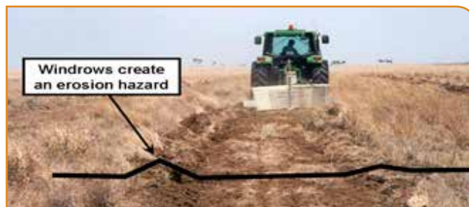
Figure 14.19: Windrows created during firebreak construction
