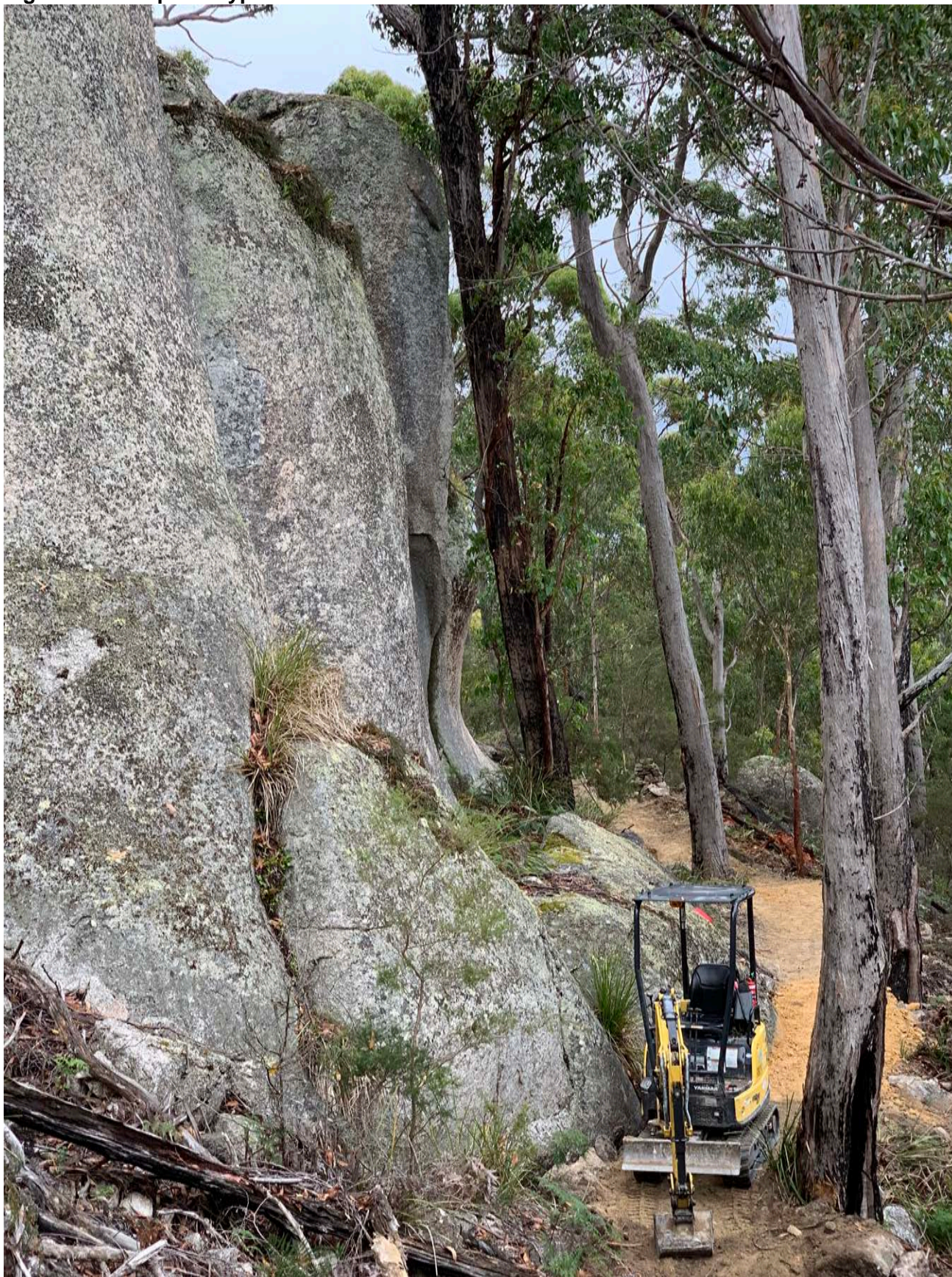
Figure 2. Example of typical mini-excavator used for trail construction
