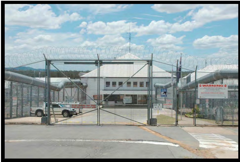
Front Gate - Borallon Correctional Centre
