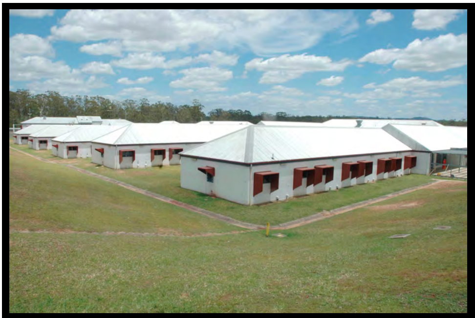
C Block - Borallon Correctional Centre
