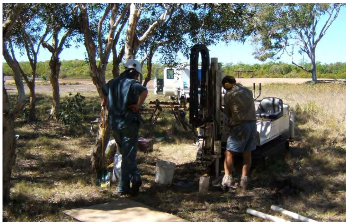
Figure 14. Installation of piezometer A, Fishing Creek.
