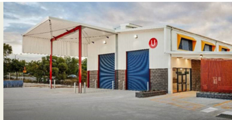
Heavy Plant Centre of Excellence at Acacia Ridge, TAFE Queensland.
