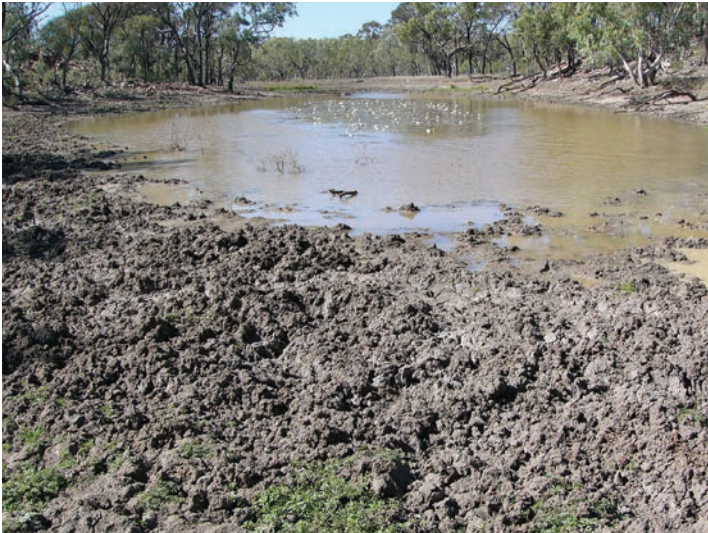
Feral pig damage to river banks
