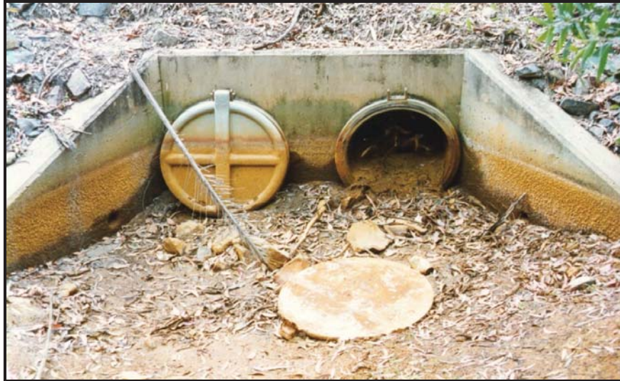
Plate 3. Acidified water from disturbed ASS attacks concrete and exposes the aggregate
