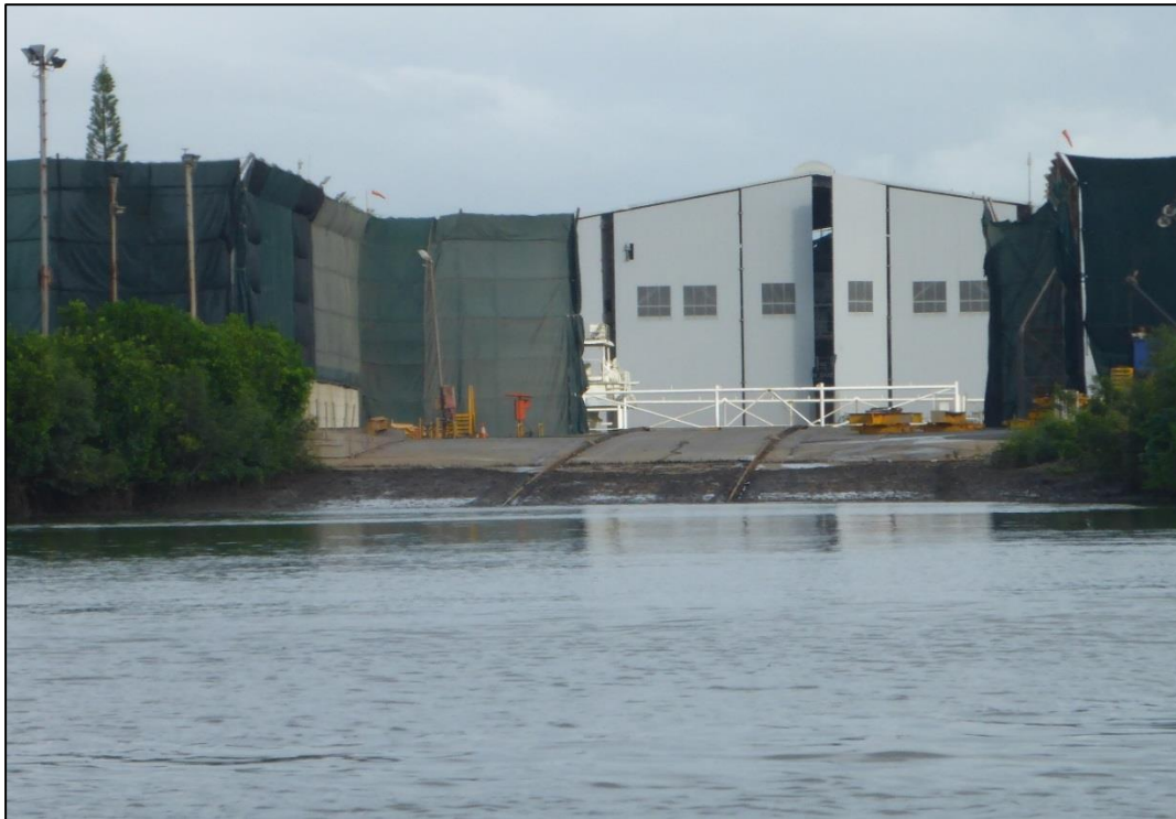
Figure 4 - BSE Cairns Slipway Showing Curve on the Slipway Tracks
