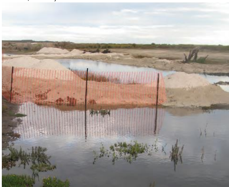
Figure A62-6: Applications of fine limestone in the Finniss River below Wally's Landing jetty to acidic waters flowing from the wetland and channel in May 2009
