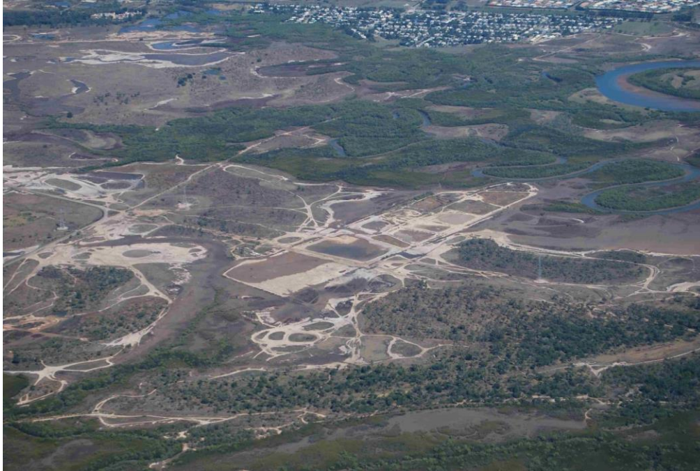
Figure A63-1: Aerial view of the site
