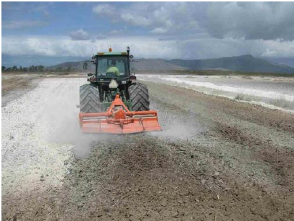
Figure A63-2: Rotary hoe mixing in surface applied aglime within excavated fill material
