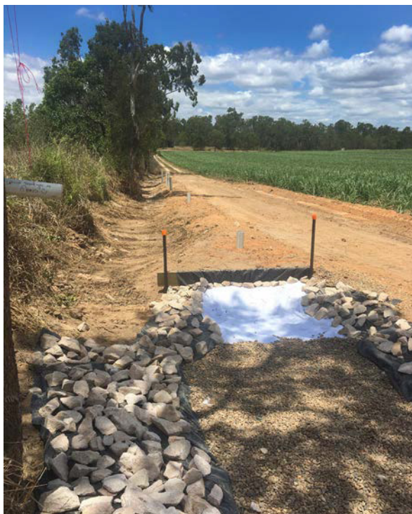
Figure 3.10 Gravel inlet pit (foreground).
