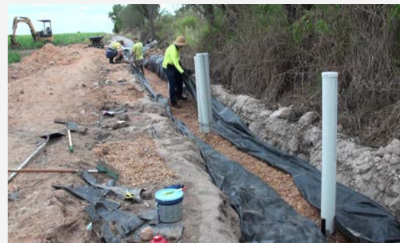
Figure 4 Bioreactor trench filled with woodchip, showing liner and piezometers.
