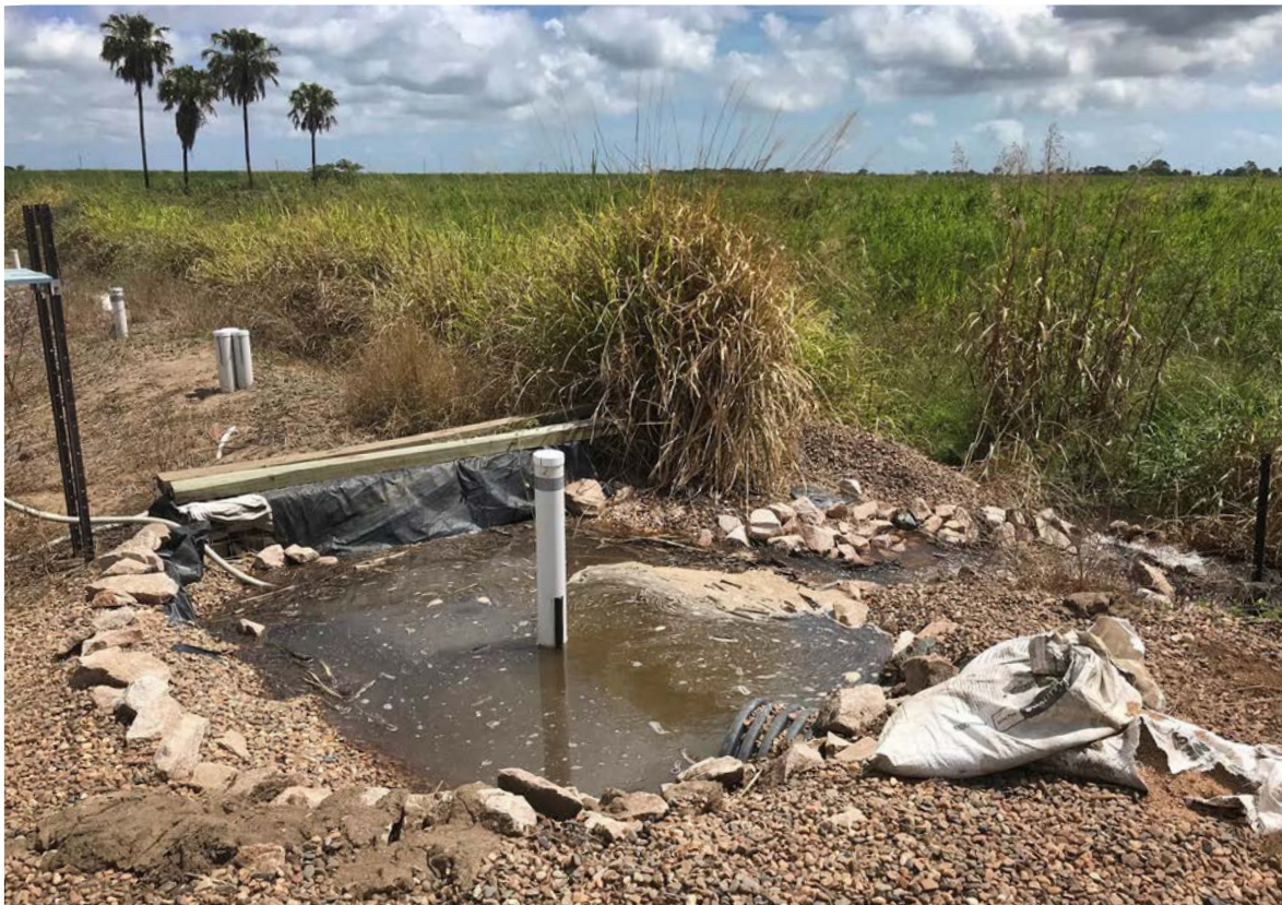
Figure 1.16 Off-line bioreactor bed installed downslope of an irrigated cane block in the Lower Burdekin.
