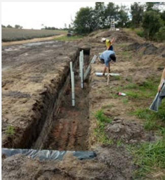
Figure 2 Construction of bioreactor walls.
