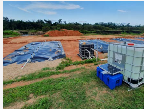
Figure 2: Woodchip bioreactor beds, showing equipment in the foreground used to add extra nitrate to test performance under different nitrate concentrations. Source: JCU
