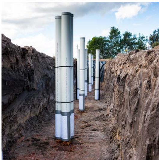
Figure 4.4 Installing a bioreactor wall for a research trial with monitoring piezometers within the wall.
