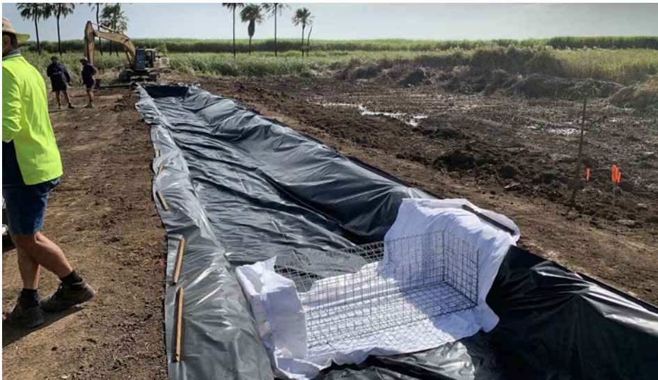
Figure 3.9 Bioreactor bed showing liner and gabion basket.
