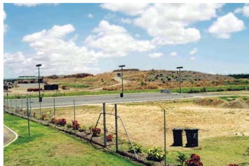
Photograph 30: Filling on tidal lands underlain by PASS at 0.8 m for the Mackay city waste disposal facility in the Pioneer River catchment area (S1)
