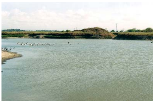
Photograph 29: Irrigation dam in the McCrearys Creek catchment excavated into acid sulfate soils at 2.0 m: note the pile of AASS spoil in the background
