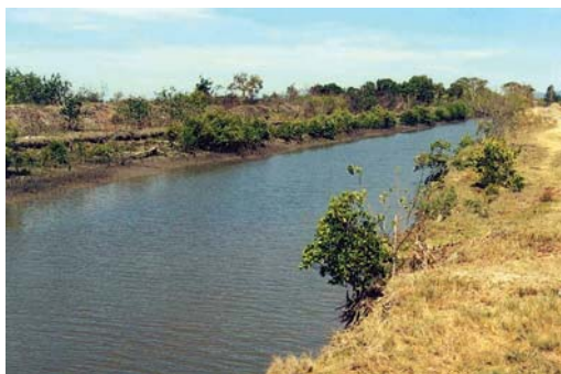
Photograph 25: South Mackay stormwater drain with ASS spoil formed into a bank on the left side of the drain
