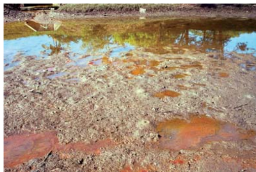
Photograph 26: Localised iron staining on the floor of a stormwater drain excavated through ASS in South Mackay
