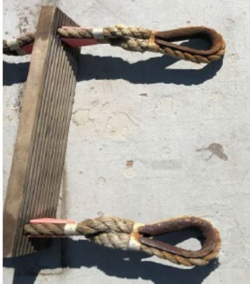
Photo 9: Example of corroded end point thimbles (Reproduced with permission from Fremantle Ports).
