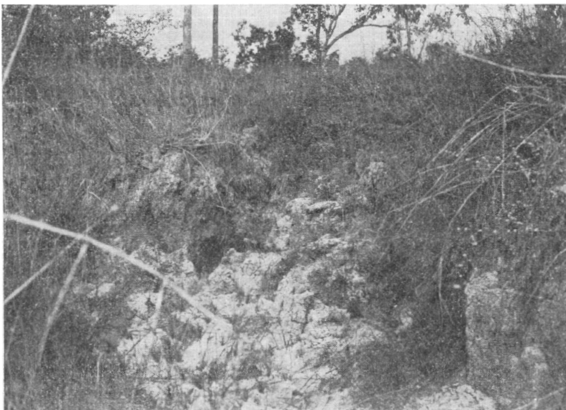
Fig. 6. Erosion of the wall of an open drain by gully head erosion. This is common where lateral surface drainage is allowed unrestricted and uncontrolled entry to the drain.
