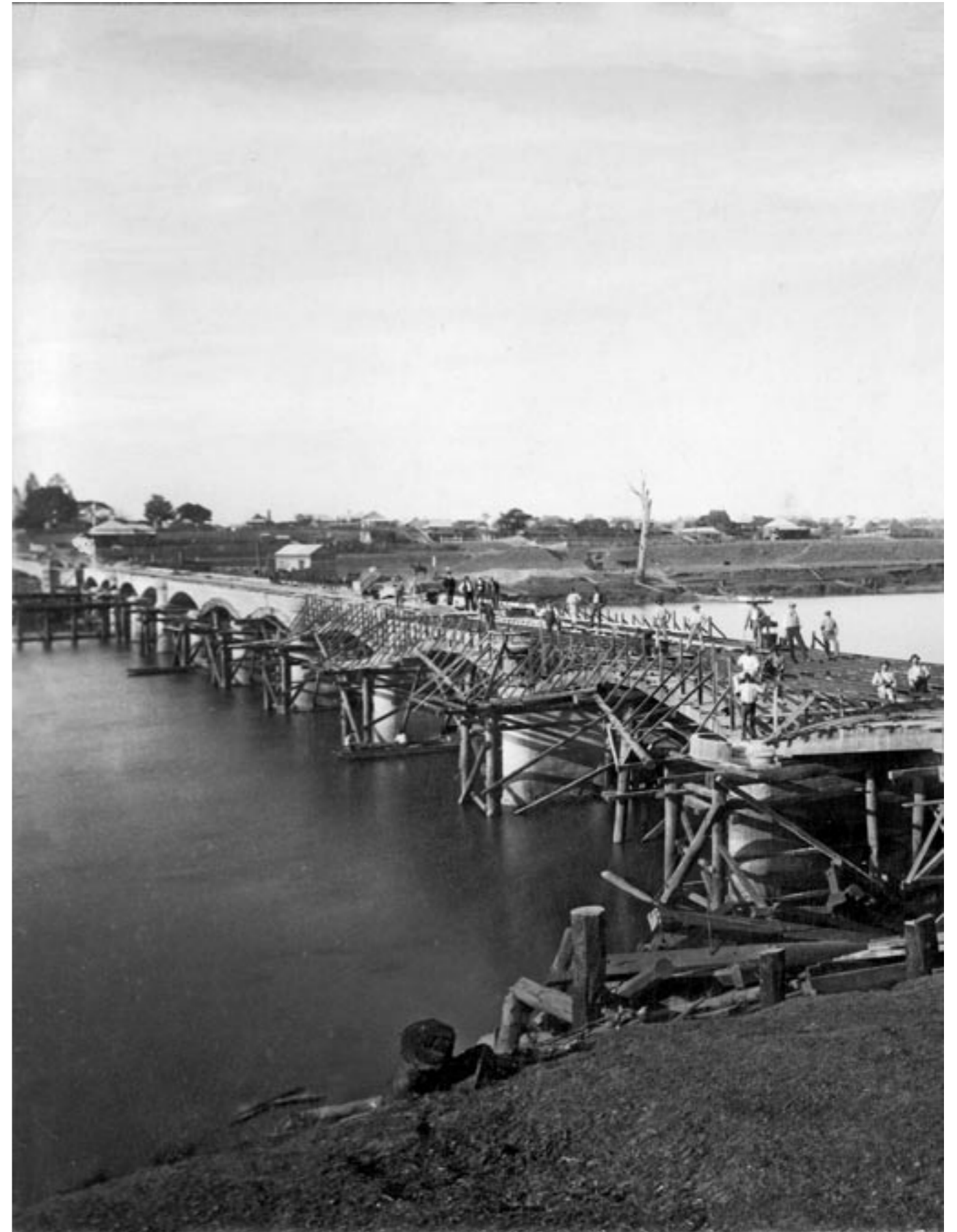
Maryborough Bridge construction, 1896 QSA Reference: PRV 14402 1 Item 2
