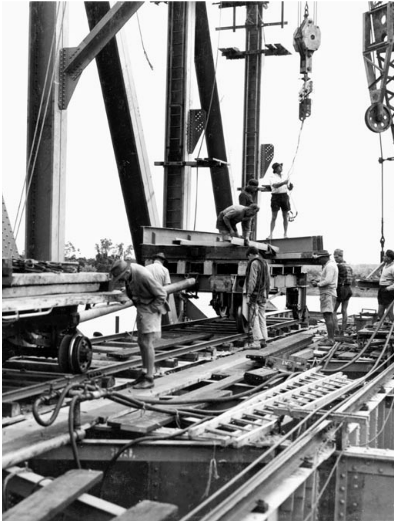
Burdekin Bridge construction, 1955 QSA Reference: SRS 194 1
