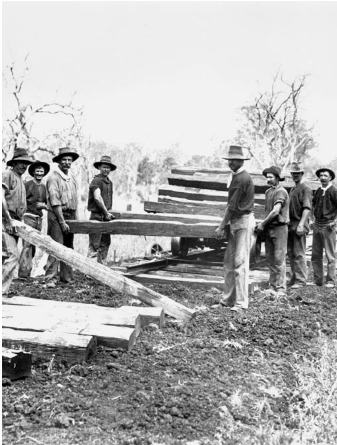
Laying railway tracks, location unknown, circa 1900 QSA Reference: SRS 189 1
