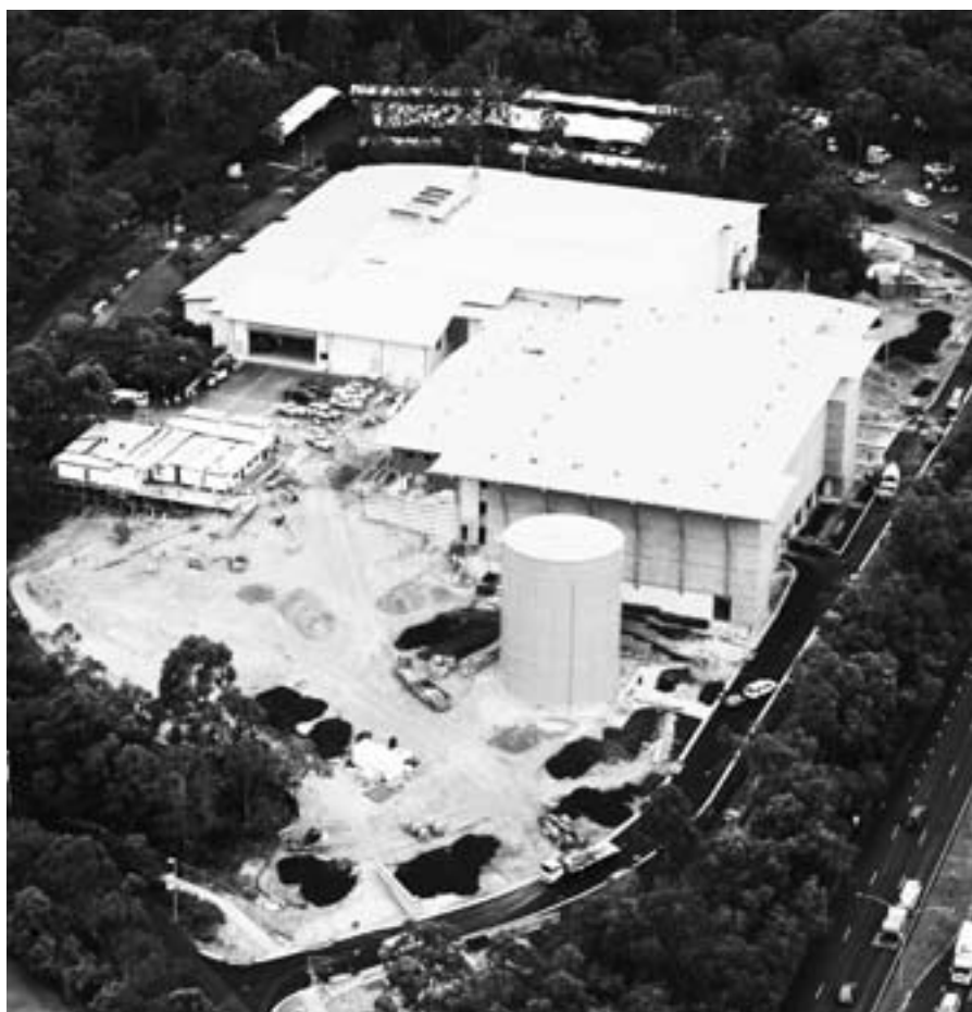
Pictured: Queensland State Archives' expansion in progress
