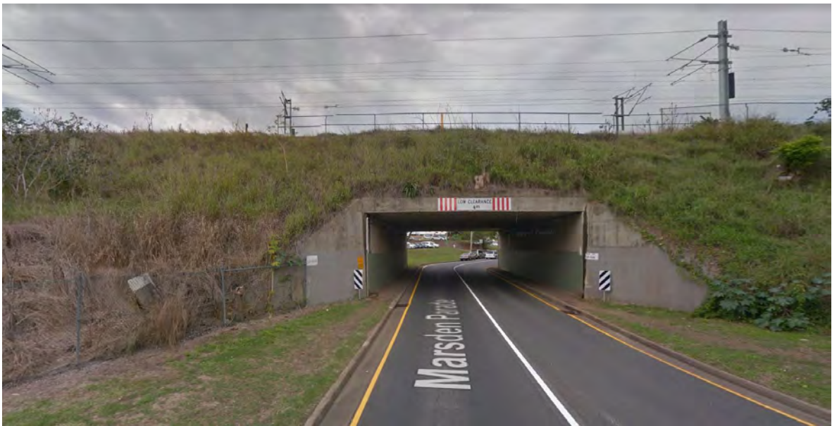
Figure 8-18 Marsden Parade Rail Underpass (source: Google streetview)
