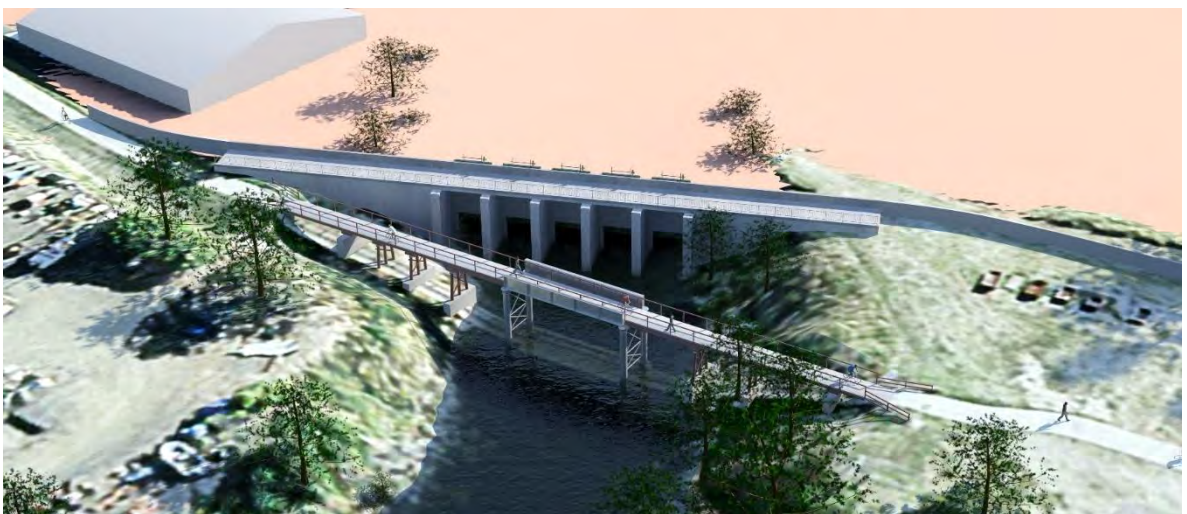
Figure 8-12 Example of sluice flood gate – concept plan, Saltwater Ck, Queensland (source: DILGP, Saltwater Creek study )
