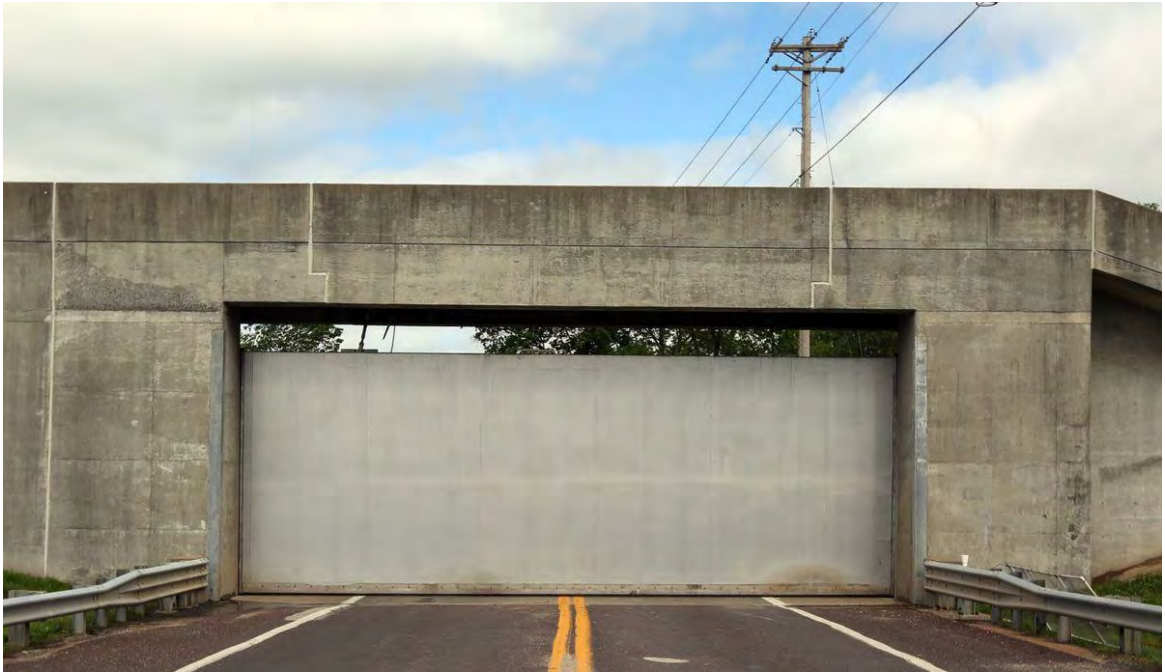
Figure 8-19 Flood gate preventing backwater inundation from the Meremac River, USA, (photo by Laurie Skrivan, post-dispatch.com)
