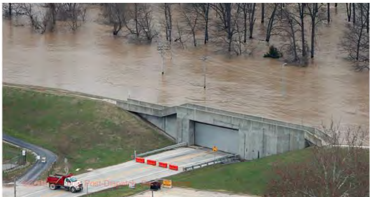
Figure 8-15 Floodgate preventing backwater inundation from the Meremac River, USA, 31/12/15 (photo by David Carson, post-dispatch.com)
