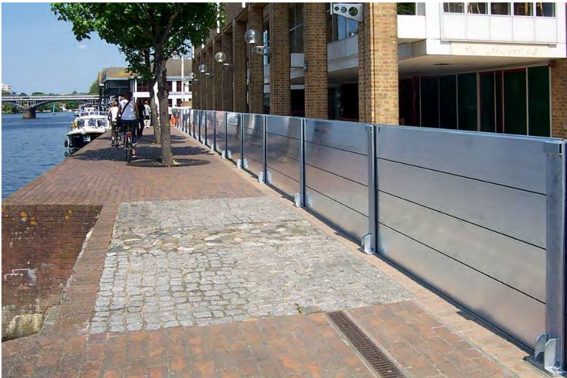
Figure 8-37 Fixed panel temporary flood barrier [ www.floodcontrolinternational.com/ ]
