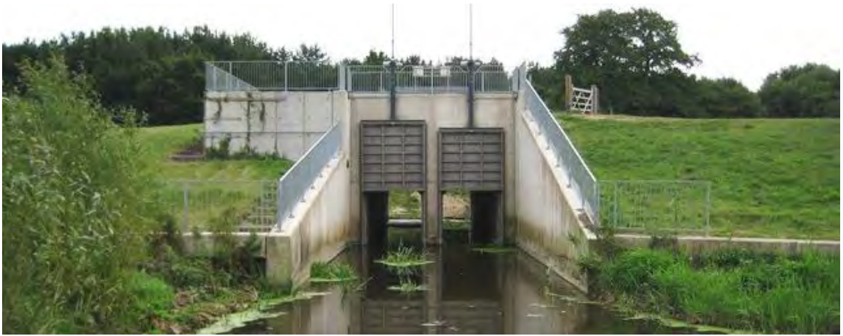
Figure 8-11 Example of sluiced flood gate, Halstead, UK (source: cc-by-sa/2.0 - © Nigel Cox - geograph.org.uk/p/1457081 )
