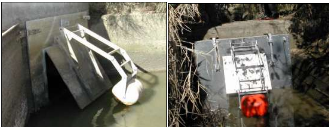
Figure 29 – Mini-gates on top-hinged floodgates
