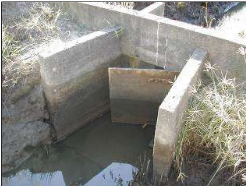
Figure 29 – Mini-gates on top-hinged floodgates
