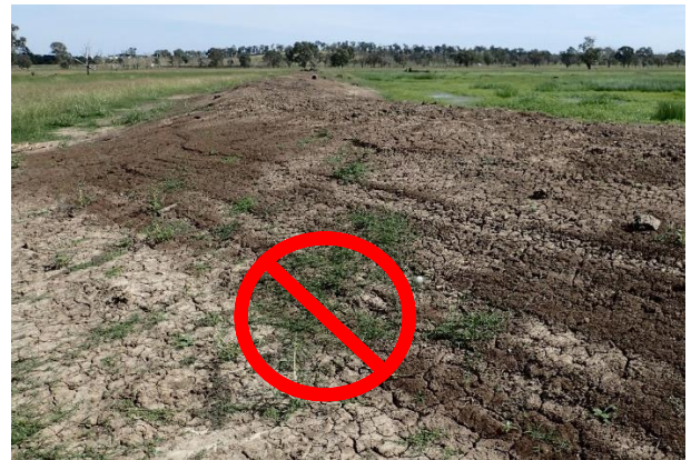
Figure 32 Vegetated areas on levee bank constructed >2 years ago Any areas on this levee bank that are currently vegetated and stable should not be considered disturbed for scoring S7.
