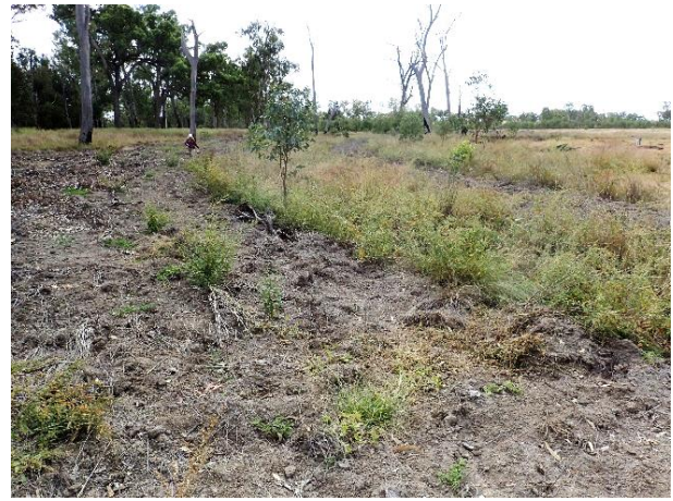
Figure 19 Bulldozer scrape around a wetland boundary. Here, we score S7 based on the % of the plot where machinery has disturbed the topsoil, leaving no protection from plants or litter.
