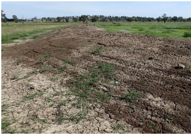
Figure 22 Levee bank. While this levee was not built recently (i.e. aerial imagery shows it is more than 2 years old), areas that remain bare were considered disturbed (i.e. unstable and/or actively eroding). Contributing factors included the replacement of topsoil with subsoil during construction (retarding plant growth) and, more recently, surface disturbance from livestock.
