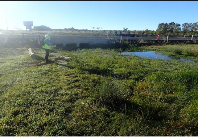
Figure 12 Stormwater outflow point from neighbouring housing estate, with water diverted into wetland (G. Borschmann, 2017). The row of small shrubs directly behind the box culvert is planted along the edge of a bio-retention pond, which holds stormwater runoff from the estate upslope. See next image (right) for aerial view.
