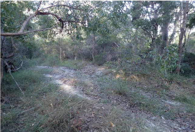
Figure 14 Drain diverting water away from road and toward a wetland (C. Johns, 2018). Spoon drains or other low gradient drains are often installed to divert water away from road edges.
