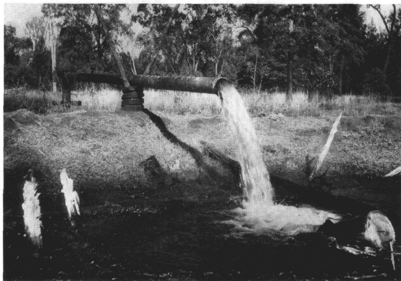
Fig. 2.—Artesian bores are a valuable source of stock water in the south-western third of the area. From the bores water is distributed to the paddocks by ditches ('bore drains').
