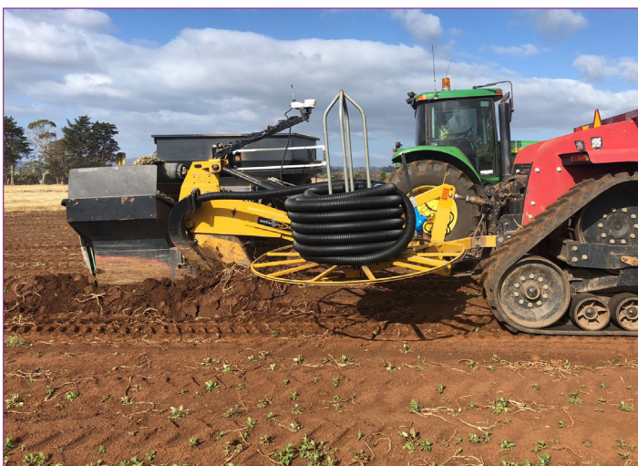
Figure 2. Subsurface drainage installation in progress at ‘Lornebrook’.
