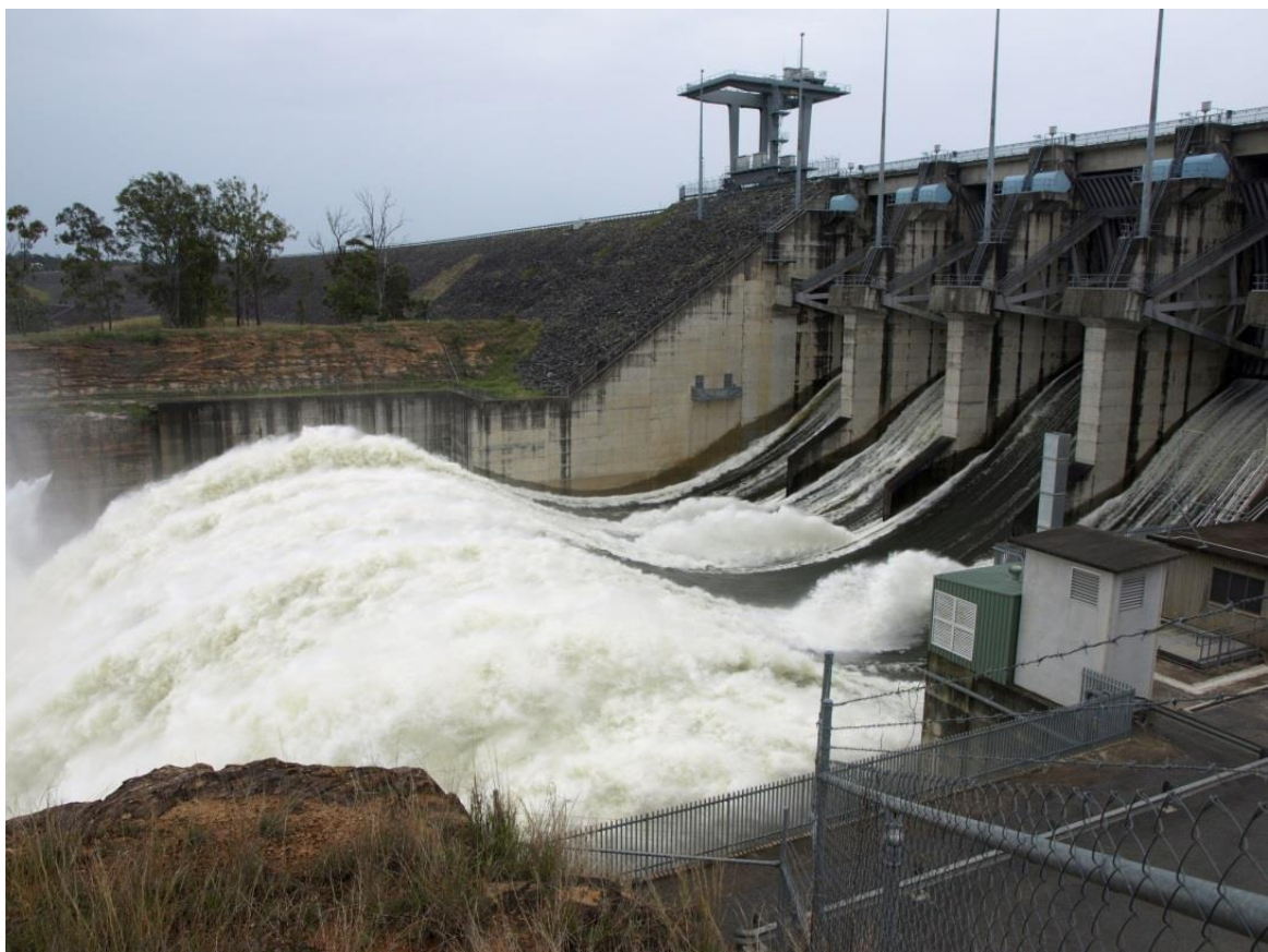
Figure 2-2 Wivenhoe Dam Spillway Releases (October 2010)
