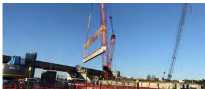
A Quickcell Super I-girder being placed on Lucinda Drive Bridge, Port Drive Upgrade Project in September 2017.
