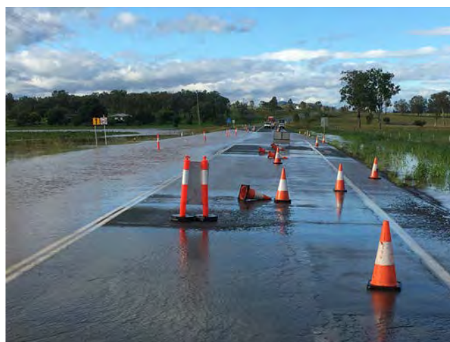
The first layer of foamed bitumen applied to the Warrill View section of the Cunningham Highway prior to the site being inundated by rainfall during Ex-TC Debbie.
