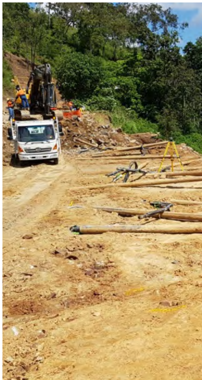
Sarina Range excavation and placement of soil nails at the main slip site.
