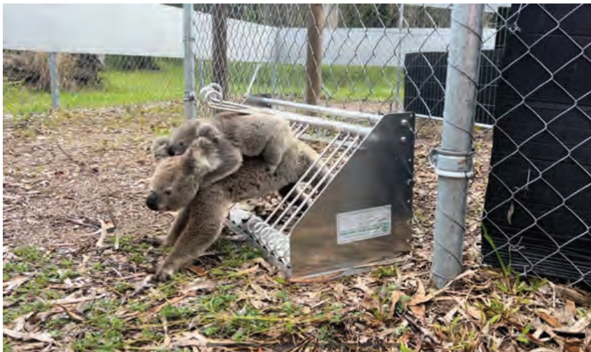
Figure 1. Female and back rider joey koalas demonstrating movement through the traditional fauna escape hatch (360mm x 1200mm)
