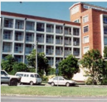
The nurses' quarters prior to demolition
