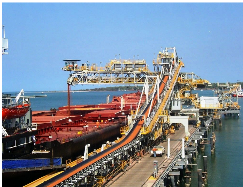
Ship loader at Weipa (courtesy NQBP)
