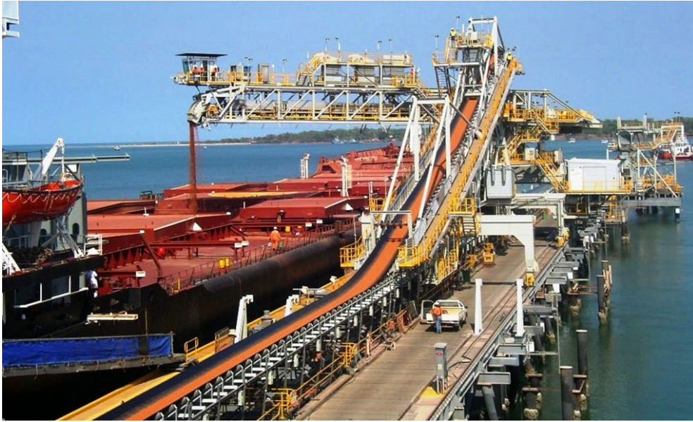
Figure 1 Ship loader at Weipa (courtesy NQBP)
