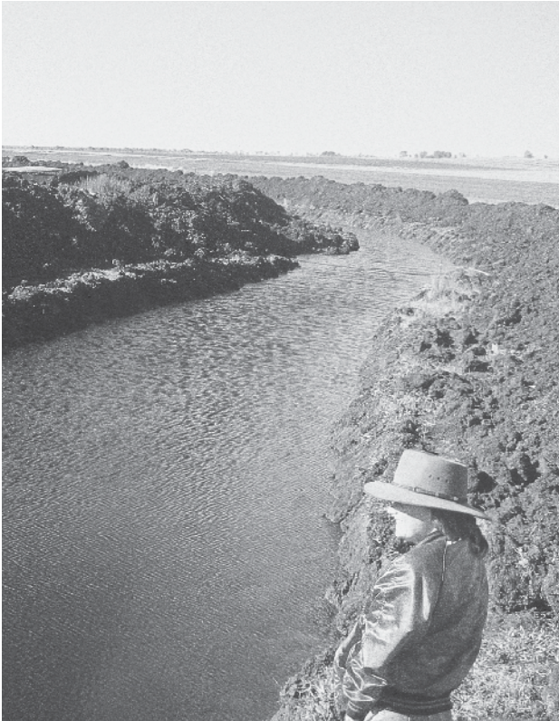
Figure 62. A groundwater interception trench in the Kingaroy district, Queensland.
