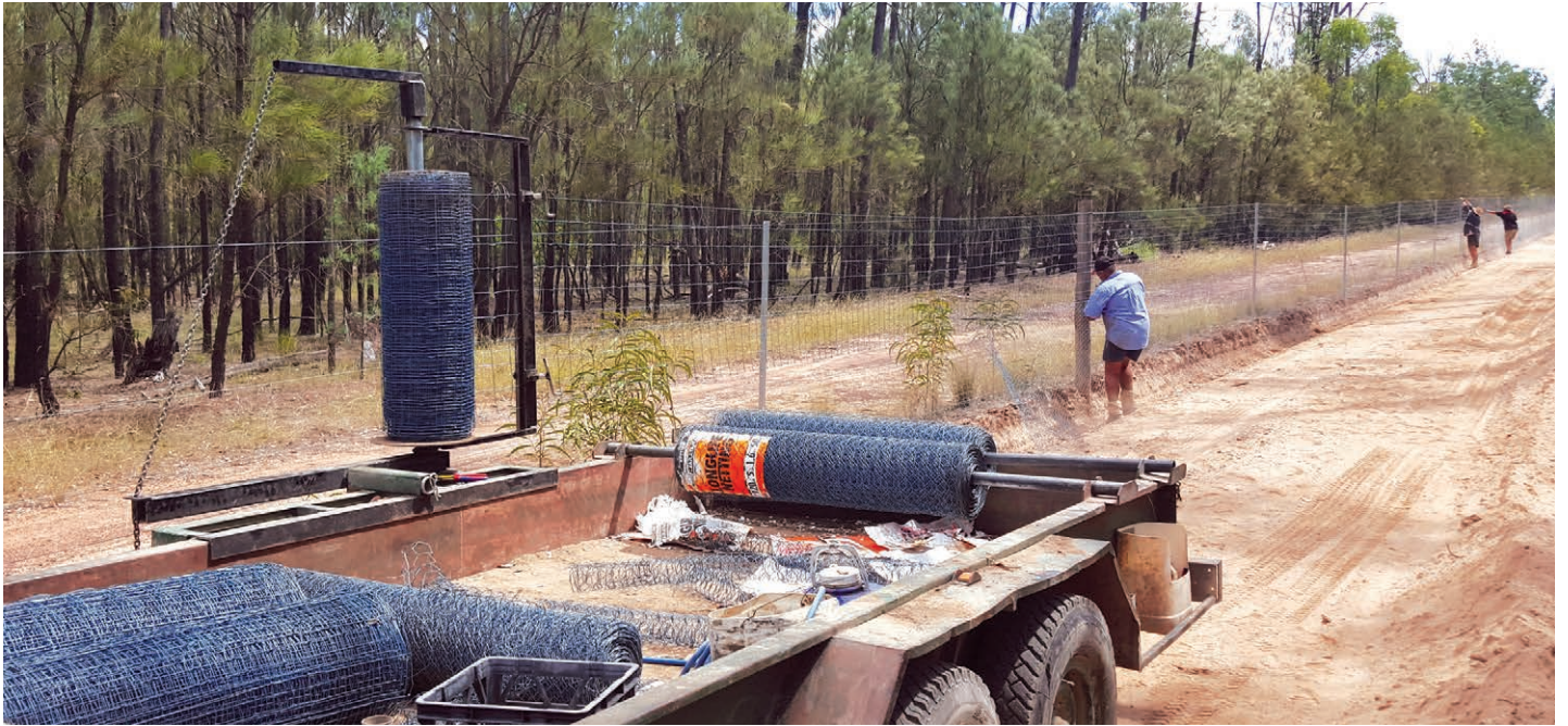
Wild dog barrier fence construction and maintenance
