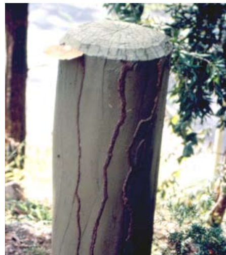
Figure 7: Microcerotermes sp. attacking painted timber decayed by the fungus Pycnoporus coccineus .
