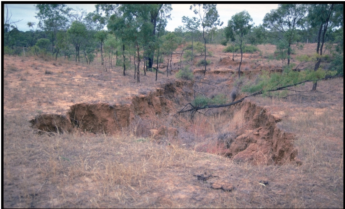
Photo 1. Erosion gully in levee bank showing that gullies can advance rapidly into alluvial plains
