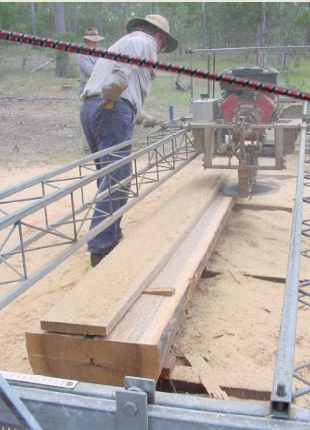
Figure 3.7 Cutting a 250 mm board required making a 200 mm cut from one side, flipping the saw over and cutting the edge board off the outside of the log and then making the final 50 mm cut.
