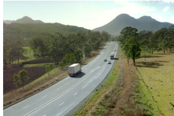
Example of wide centre lines on [road]
