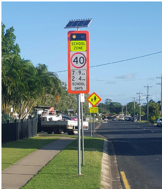
In April this year flashing school zone signs were installed in the Grevillea Street school zone at Kawungan State School, Hervey Bay
