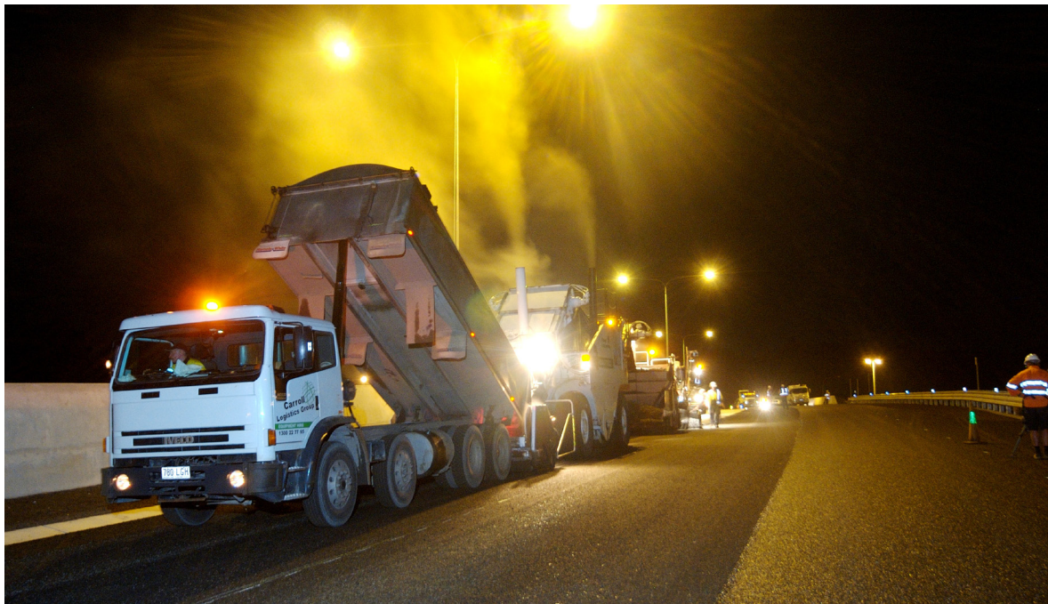
Night work upgrades to the Gateway Motorway
