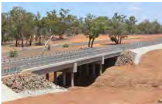
New bridge over Angellala Creek
