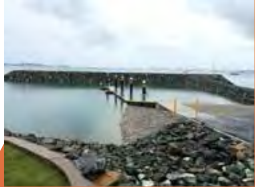
Whisper Bay floating walkway
