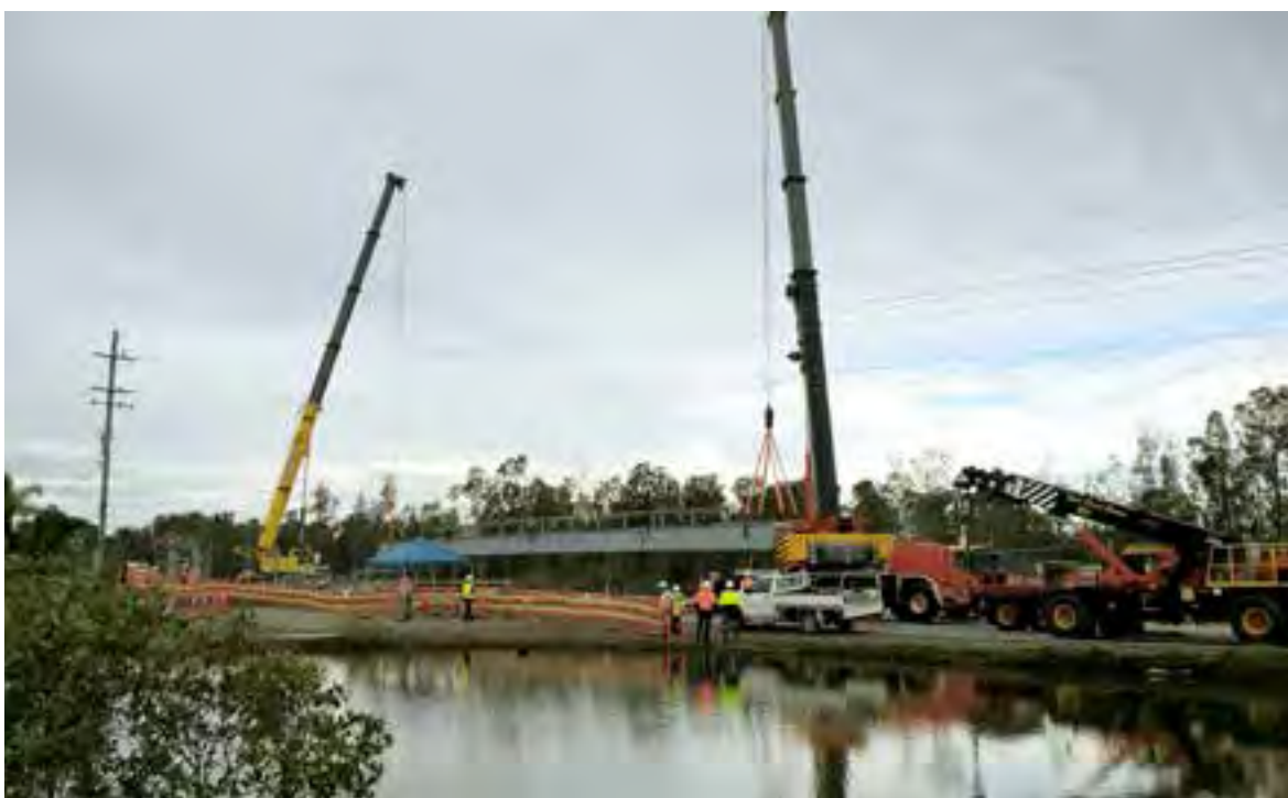
Behm's Creek bridge replacement
