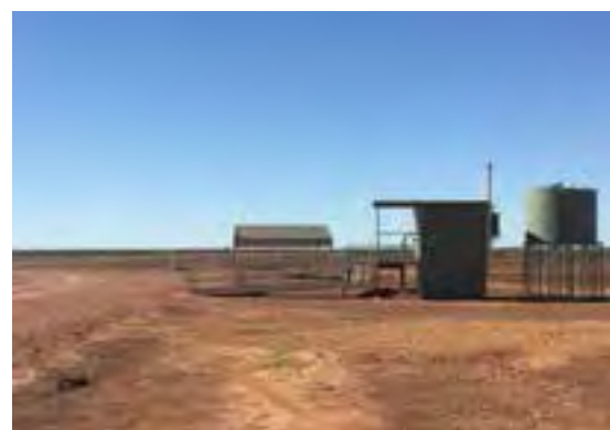
Middlemount Road, Dysart (above) and Diamantina Development Road, Monkira (about 270 kilometres north-east of Birdsville) (below) are two of the heavy vehicle rest areas reviewed during the audit
