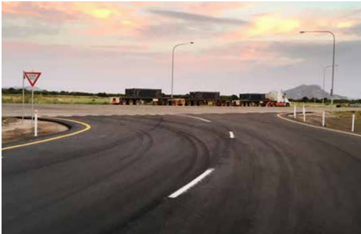
AWP road train decoupling pad, Townsville Port Road
