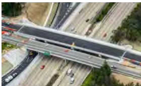
Exit 54 new bridge
