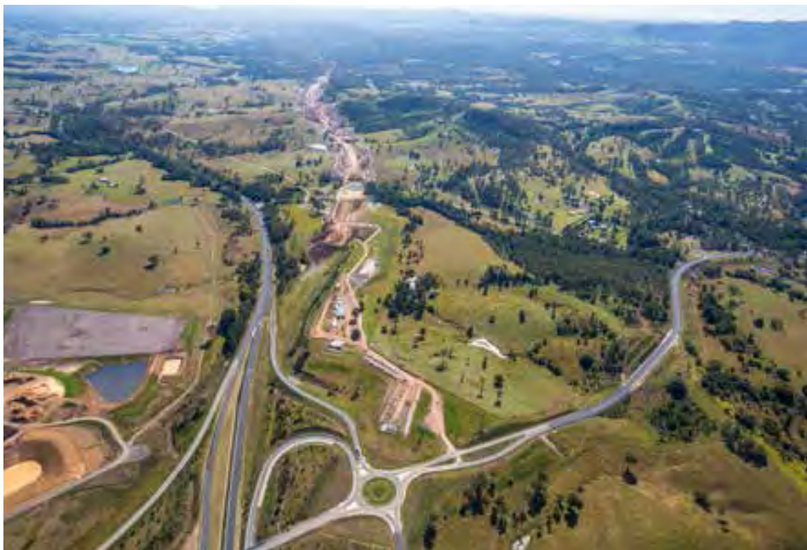
Progress on Cooroy to Curra Section C – looking north from Traveston interchange (June 2016)
