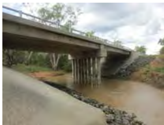
Native Companion Creek Bridge
