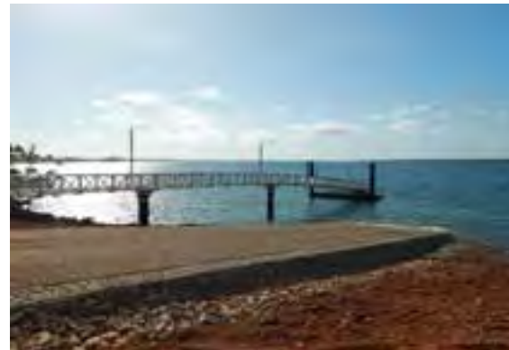
Weipa new boat ramp and pontoon
