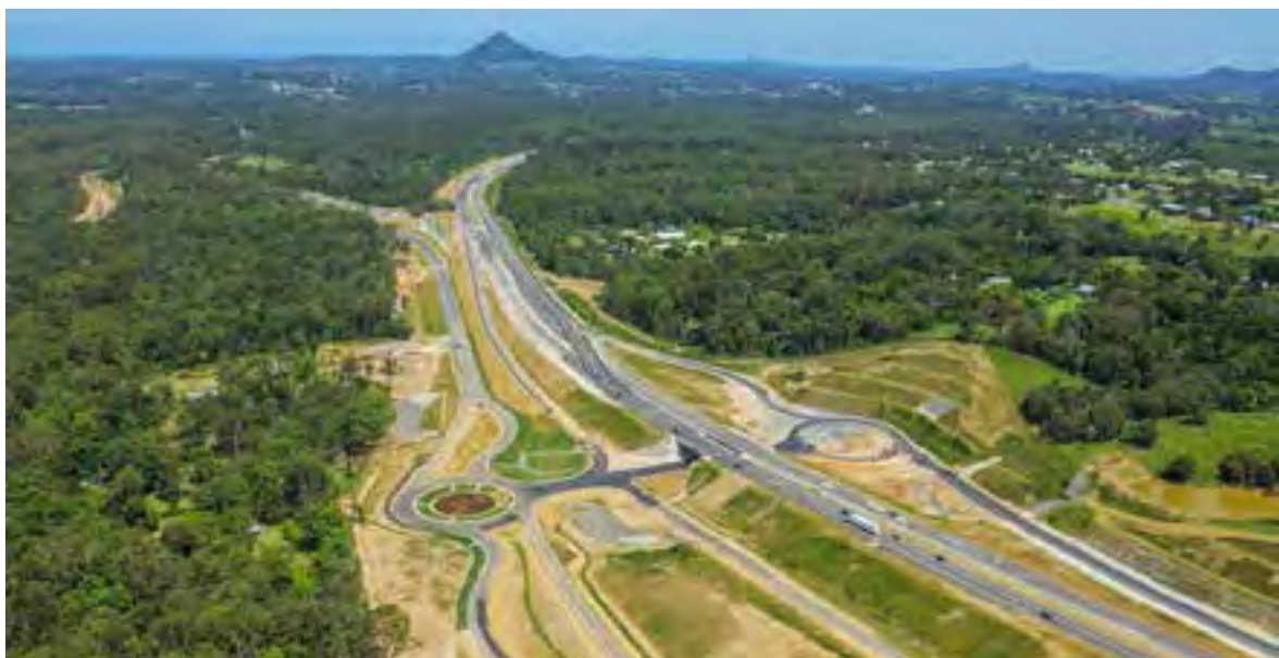
Cooroy to Curra (Section A) looking south, December 2015
