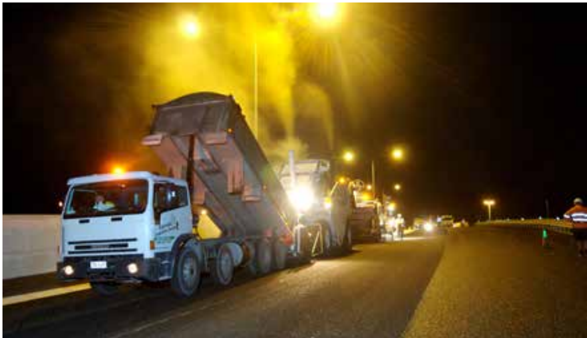
Night work upgrades to the Gateway Motorway
