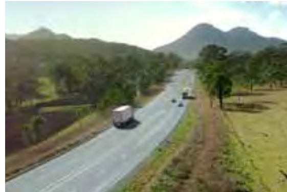
Example of wide centre lines on [road]
