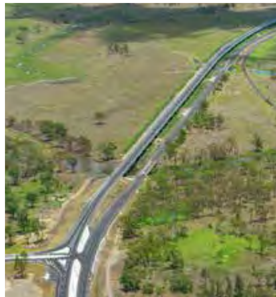
Yeppen South Bridge, an elevated crossing of the floodplain on the Bruce Highway south of Rockhampton
