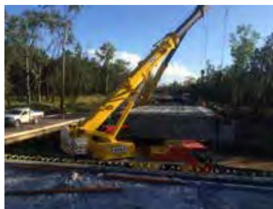
Wambo Creek Bridge
