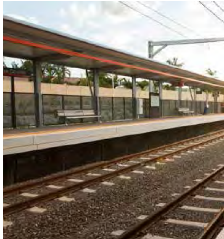
Murrumba Downs station
