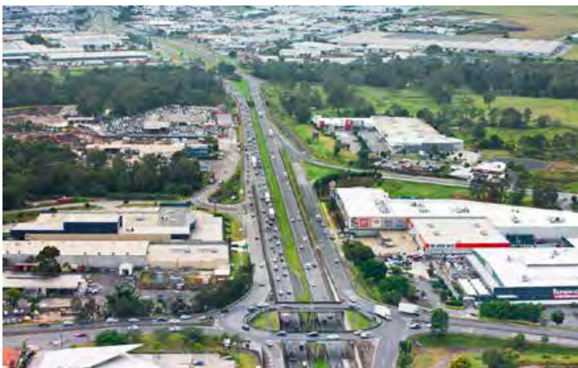
Ipswich Motorway upgrades
