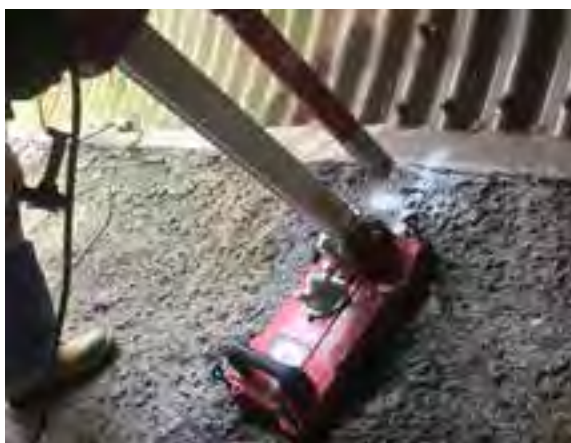
A new coring process for steel culvert inspections that will save time, equipment and resources. Left: core drilling, Right: inspection and testing.
