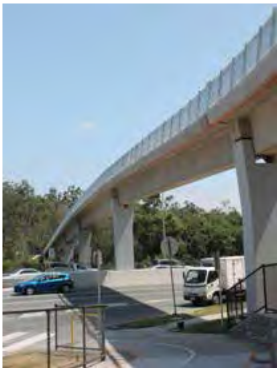
Centenary cycleway – Moggill Road Cycle Bridge
