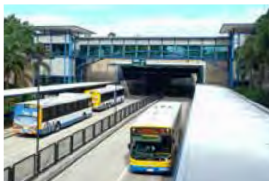
South East Busway – Buranda Station
