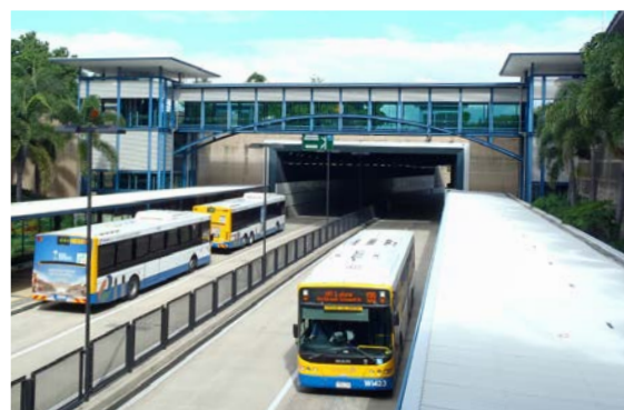
South East Busway – Buranda Station
