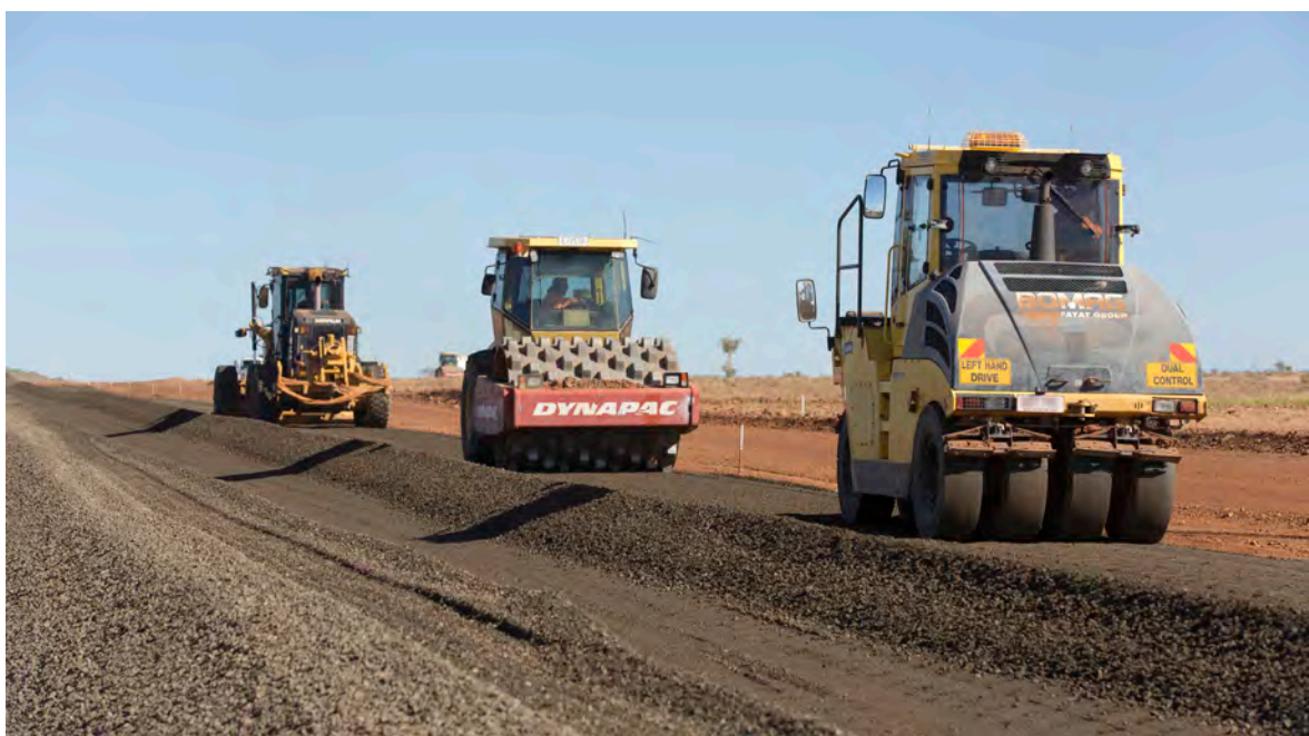
Plant in operation on the Cloncurry-Dajarra Road (Cloncurry-Duchess) as part of the Western Roads Upgrade Program
