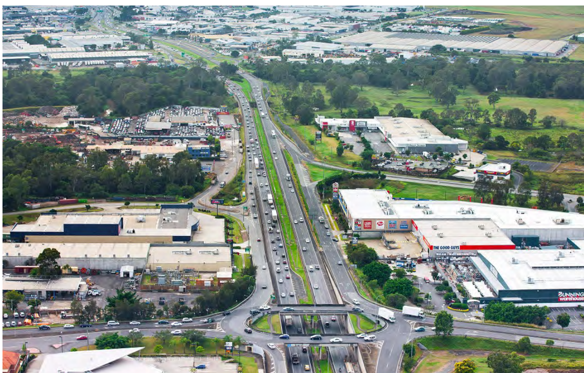
Ipswich Motorway upgrades
