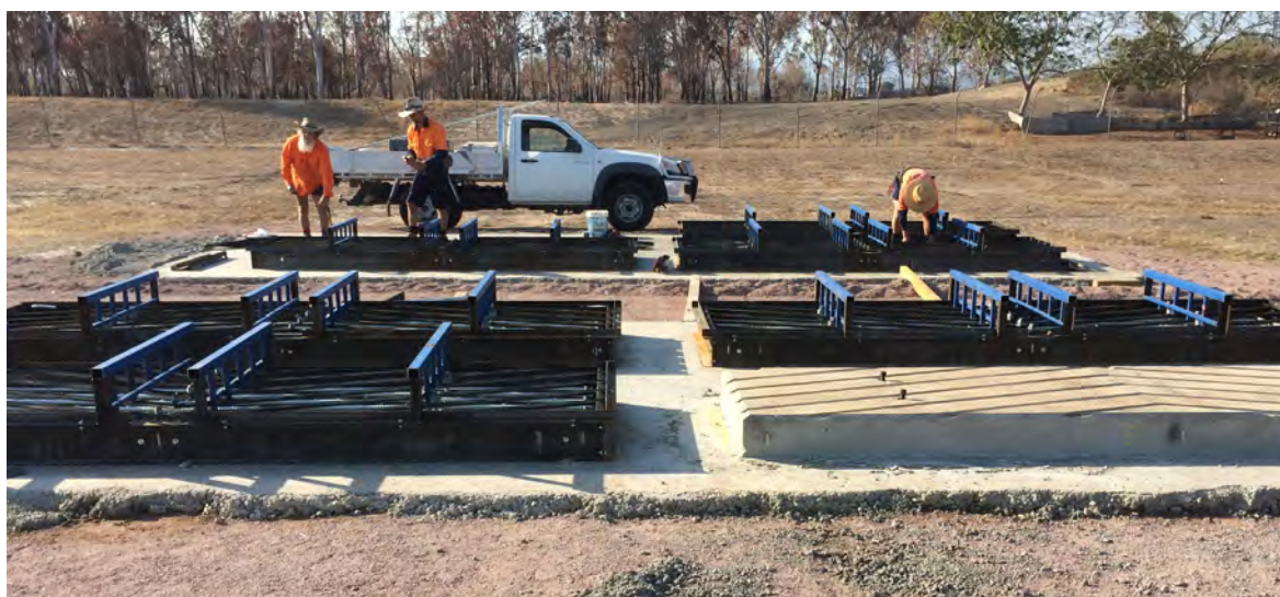
Precast structures manufactured for the reconstruction of Wallace Landing boat ramp and the BP Home Hill access reconstruction by the department saved money and time.
