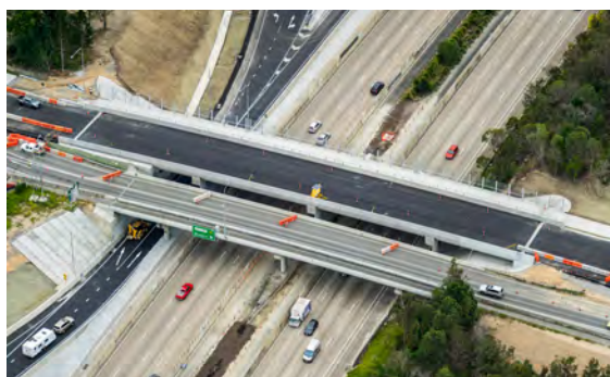
Exit 54 new bridge
