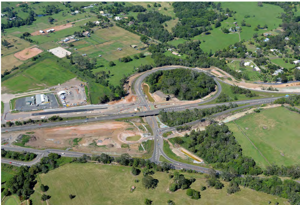
Aerial photo of works underway to upgrade the Cooroy southern interchange
