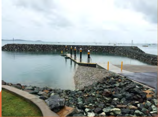
Whisper Bay floating walkway
