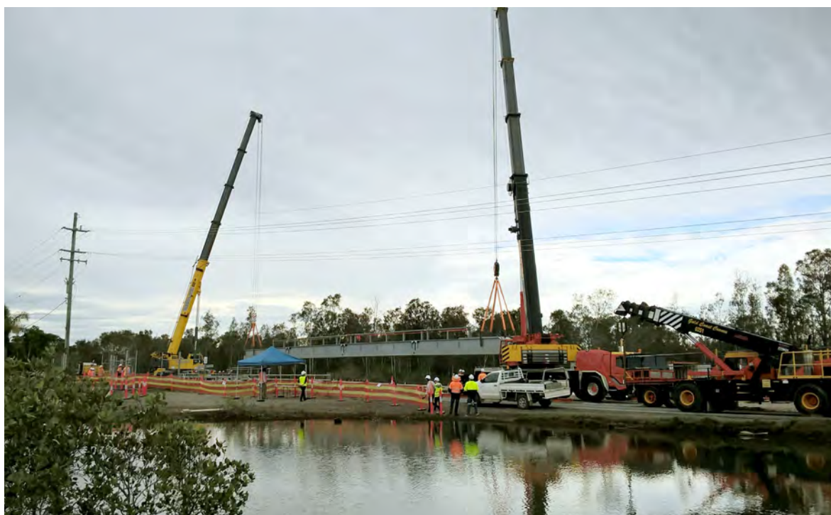
Behm's Creek bridge replacement
