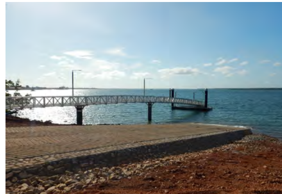
Weipa new boat ramp and pontoon
