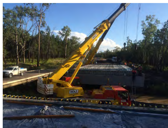
Wambo Creek Bridge
