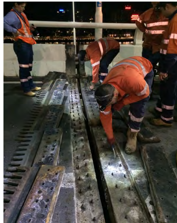
New work practices including the custom design tooth to clean bridge joints.
