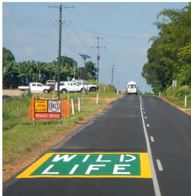
Installation of Vehicle Activated Signs for cassowary alerts.
