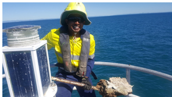
Prathee enjoying work on a structure in Main Channel, Moreton Bay, during his time with MSQ.
