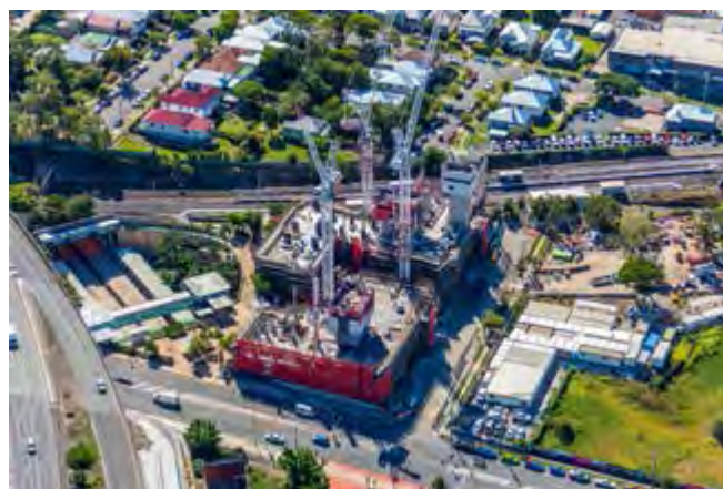
Buranda transit oriented development, Stage 1 under construction in April 2017
