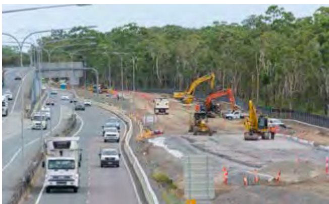
Gateway Upgrade North – Deagon Deviation widening.
