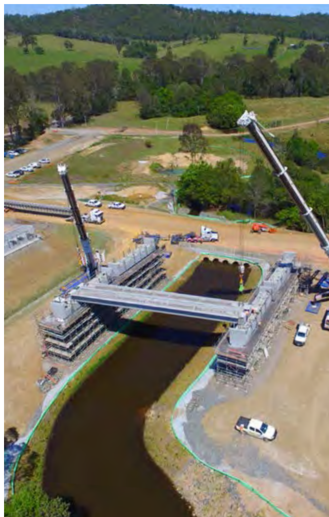
Bruce Highway – Cooroy to Curra (Section C) Traveston Bridge Girder placement.
