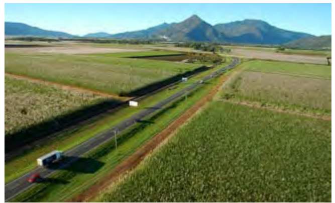
Aerial view of Bruce Highway in far north Queensland.
