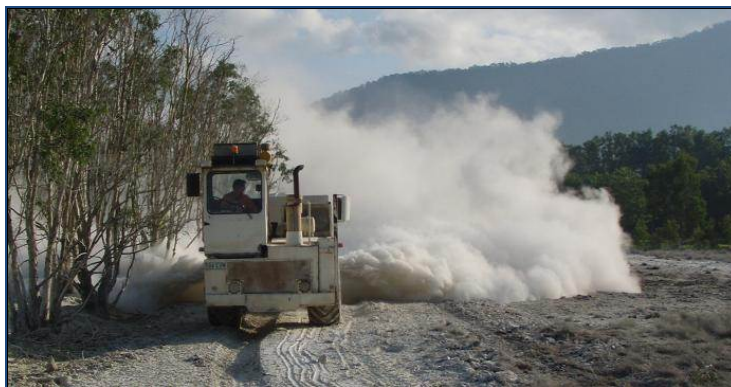
Figure 1 – Lime application for treatment of acid sulfate soils.
